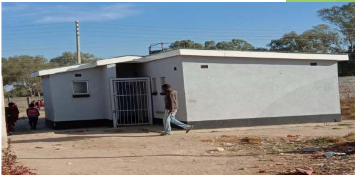
Chitungu council toilet built in Ward 4, Epworth using devolution funds
