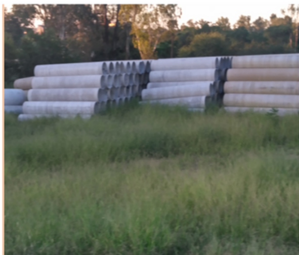
Pictures showing 750 mm asbestos cement pipes for the Mucheke Trunk sewer, and some of them broken and vandalized.
