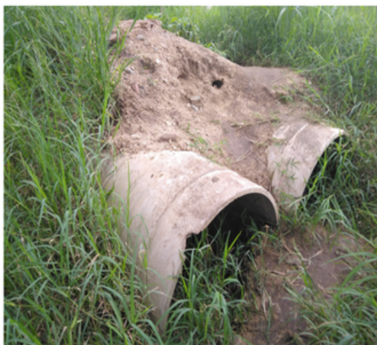
Pictures showing 750 mm asbestos cement pipes for the Mucheke Trunk sewer, and some of them broken and vandalized.
