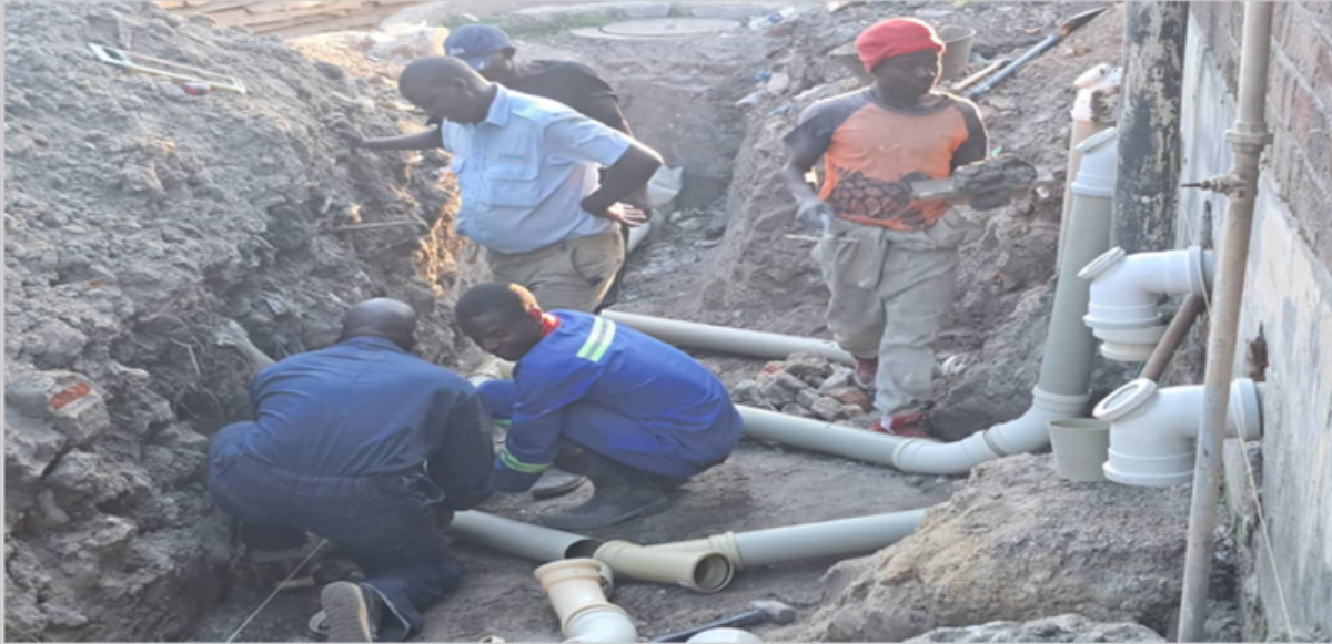
Image: Council workers laying sewer pipes
