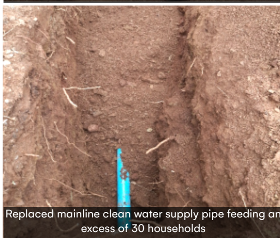
Bulawayo city council workers replace burst 1992 water pipes in Ward 3
