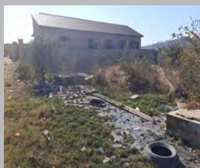
Figure 16: sewage flowing into residential areas in Izayi Park, Zvishavane
