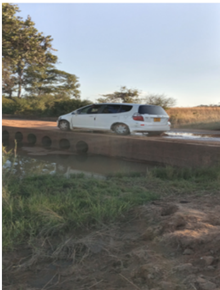
Shallow Bridge in ward 13
