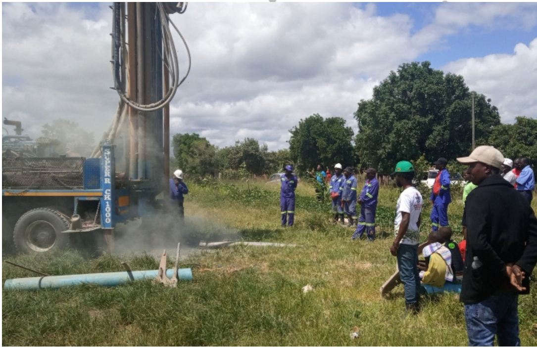
One of the boreholes drilled by Bikita RDC in Bikita South's Ward 1 recently at a cost of US$9000
