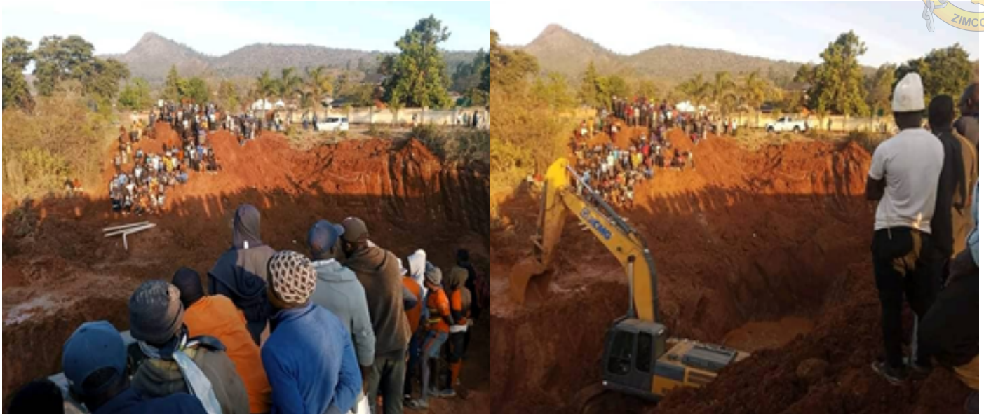
The above pictures show the mining site along the Mutare River where two people are said to have died and their bodies are not yet recovered.
